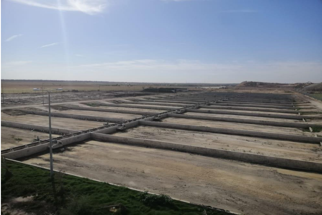
Drying Beds Cleaned from Dried Sludge in December 2021
