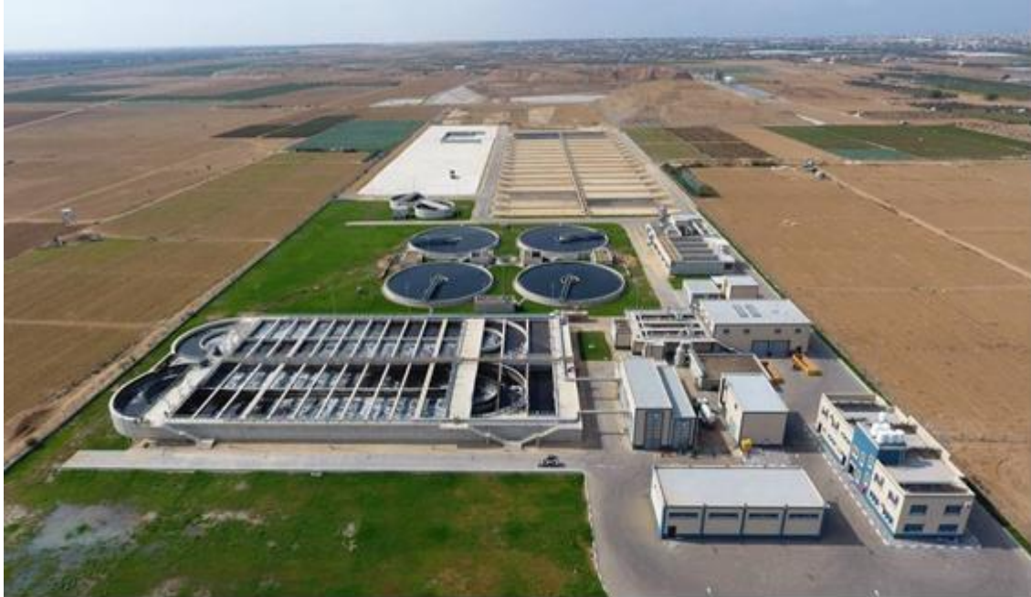
General Overview for KY WWTP Filled after Being Filled with Wastewater in September 2019
