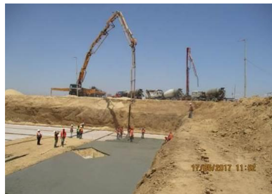
Starting Casting Reinforced Concrete for Admin Building and Plain Concrete for Aeration Tank on 17 May 2017
