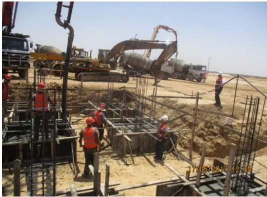
Starting Casting Reinforced Concrete for Admin Building and Plain Concrete for Aeration Tank on 17 May 2017
