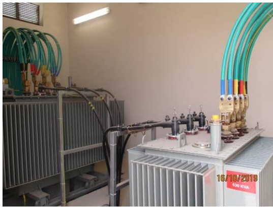
Installed Electrical Poles, Cables and Transformers of the Main Electrical Line for KY WWTP
