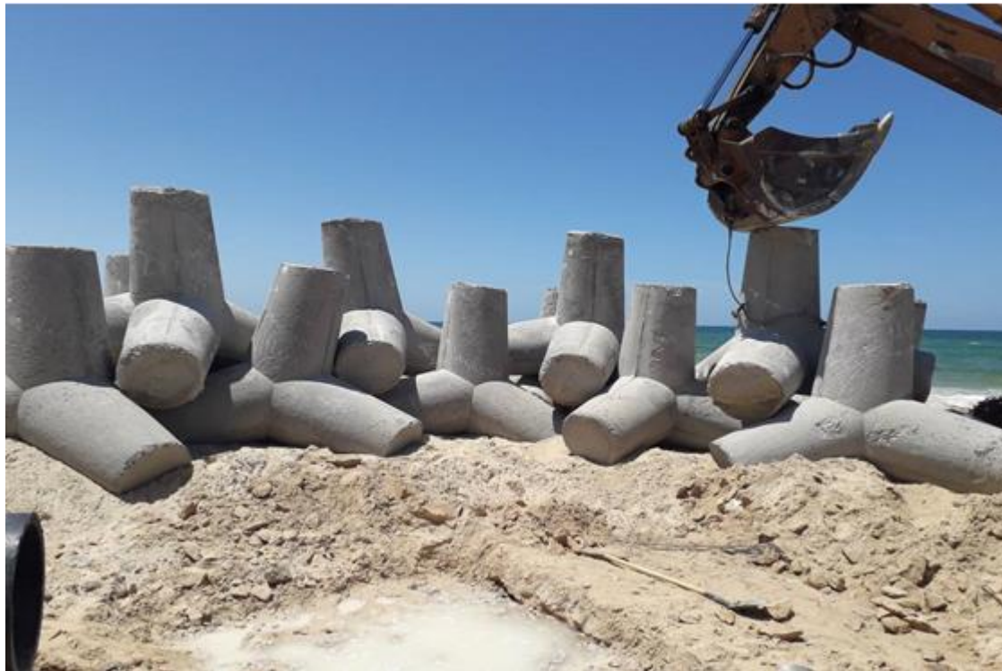
Installation of HDPE Pipes and Interlocking Blocks Tetrapod Shape for Sea Outfall for the Effluent Pressure Lines (CMWU Package) up to Completion in June 2020
